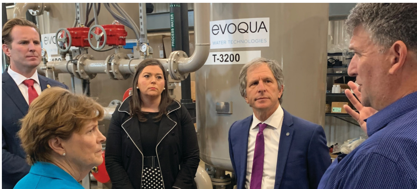
EPA Region 1 Administrator and PFAS Executive Council co-chair David Cash tours a drinking water treatment facility in Portsmouth, New Hampshire, with Senator Jeanne Shaheen and community leaders.
